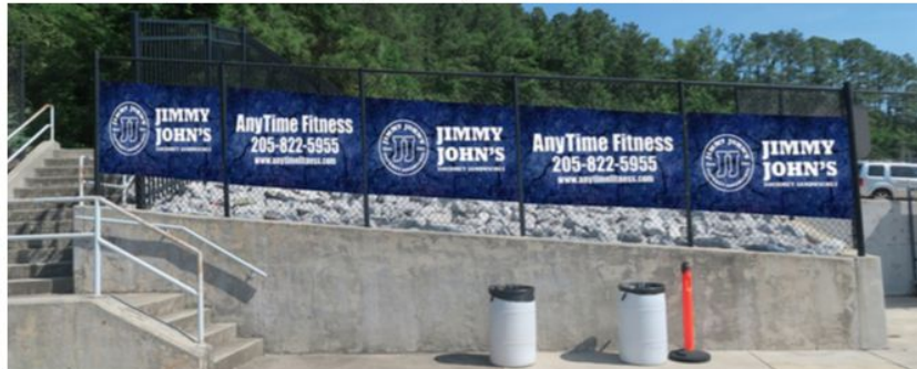
68" x 60" Parking Lot Fence Facing Stadium (Fence behind rocks)
